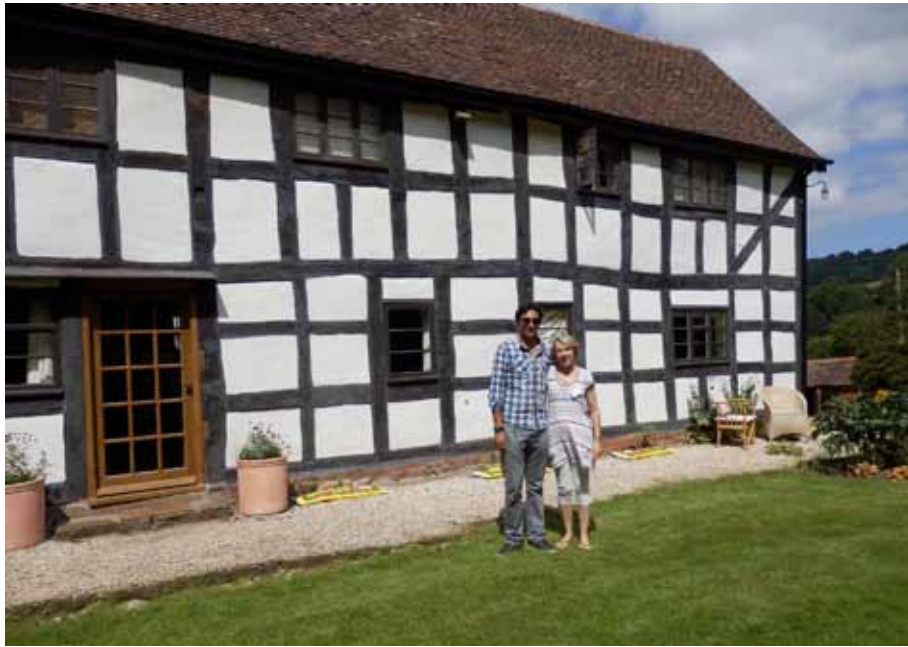
Ham Bridge House
